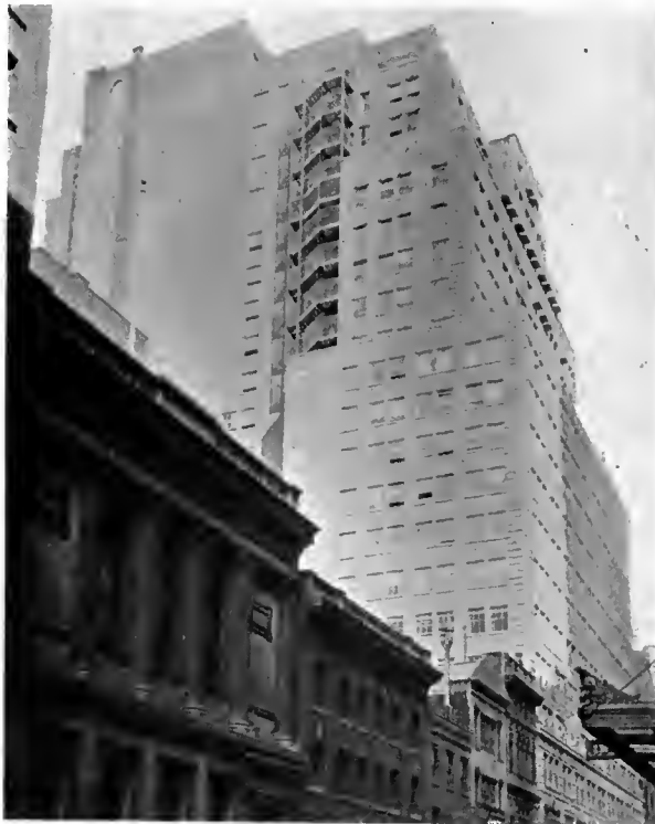
FIG. 8. NATIONAL ASSOCIATION BUILDING, WEST FORTY-THIRD STREET, NEW YORK
